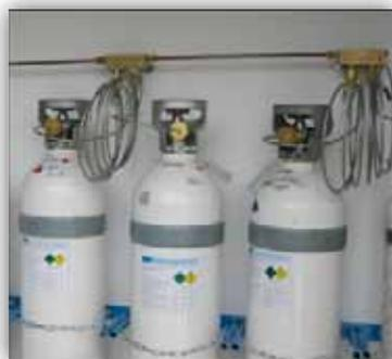
1) Central de gases: tubo flexível, conector, tubo colector.
